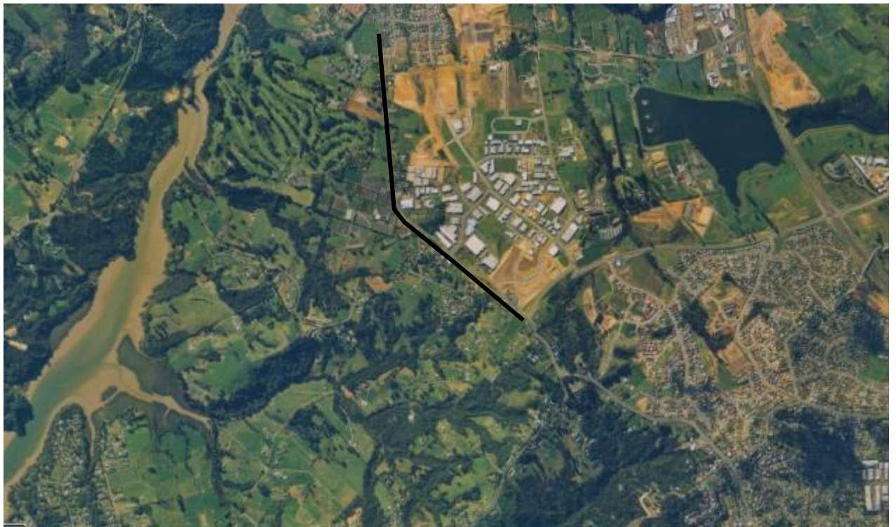
Figure 12. 1996 aerial of the project area within Albany and Rosedale, showing extensive earthworks being undertaken along the eastern side of Albany Highway (shown in black) and within Rosedale Park (towards the upper right-hand corner). Source: Auckland Council GIS 2014
