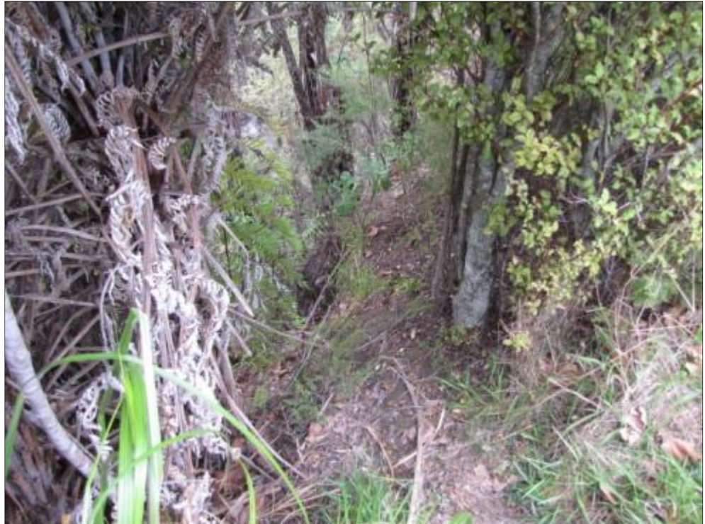
Figure 64. Exposed soils along river bank at North Shore Golf Club end of alignment
