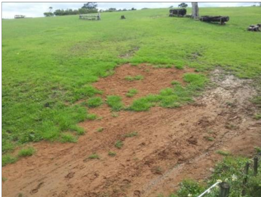
Figure 56. Exposed soils within South Wainoni Park
