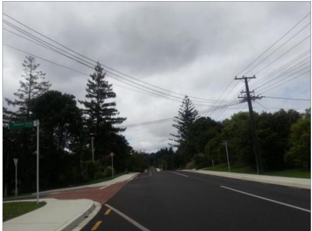
Figure 51. Looking south down proposed alignment on Tauhinu Road
